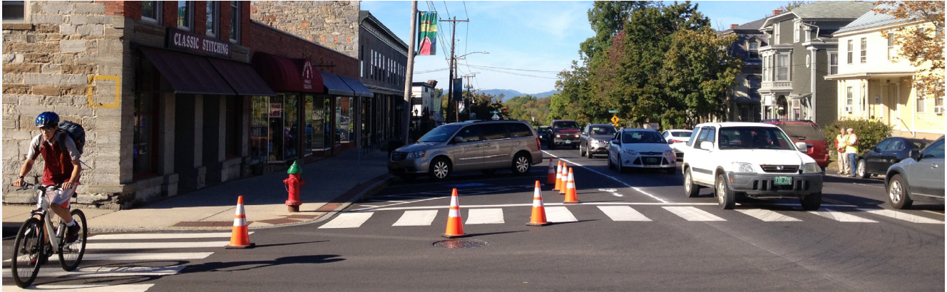
Temporary 'bulb-out' / curb extension at the corner of Green Street and Main Street as part of the Community Event demonstration projects in September of 2015.
